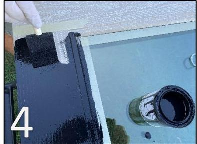
8. Wait for the base coat to cure to a tack free finish before applying the TruCoat – Grain. This typically takes 5 to 10 minutes depending upon temperature and humidity.
